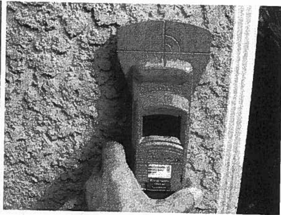
Masonry wall are steel reinforced.
