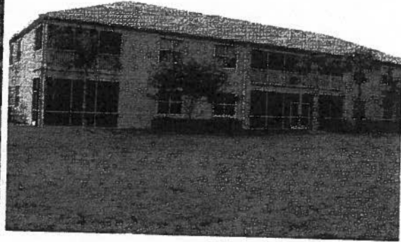
Rear elevation of building.
