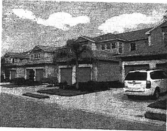
Front elevation of building.
